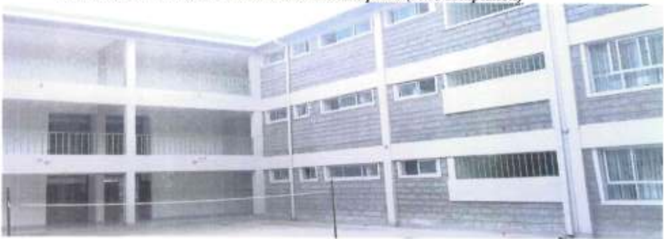
Picture 3: Library Block Under Construction (Front Elevation)- 55% completion
