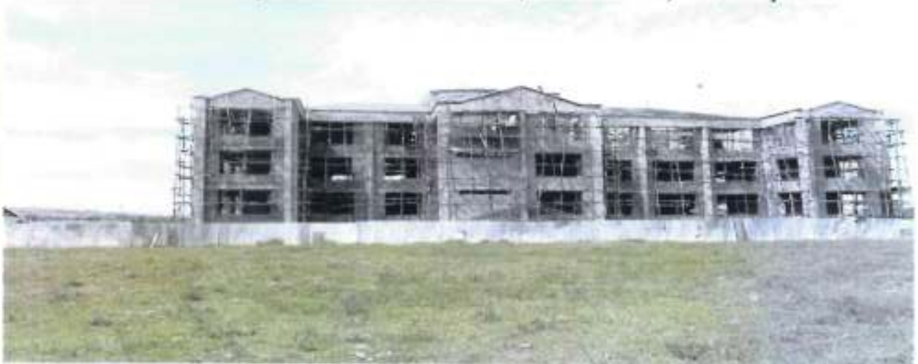
Pictures 4: Students Multipurpose Hall under construction- 90% completion
