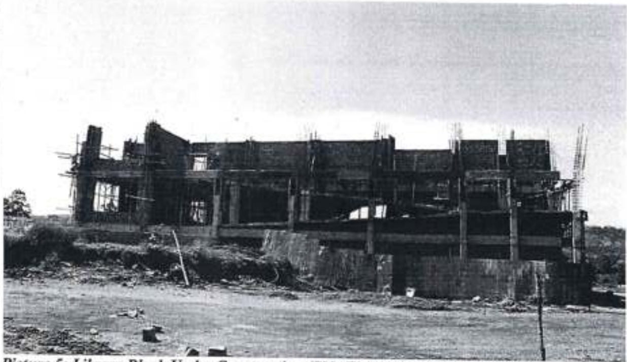
Picture 5: Library Block Under Construction (Side Elevation)- 40% completion
